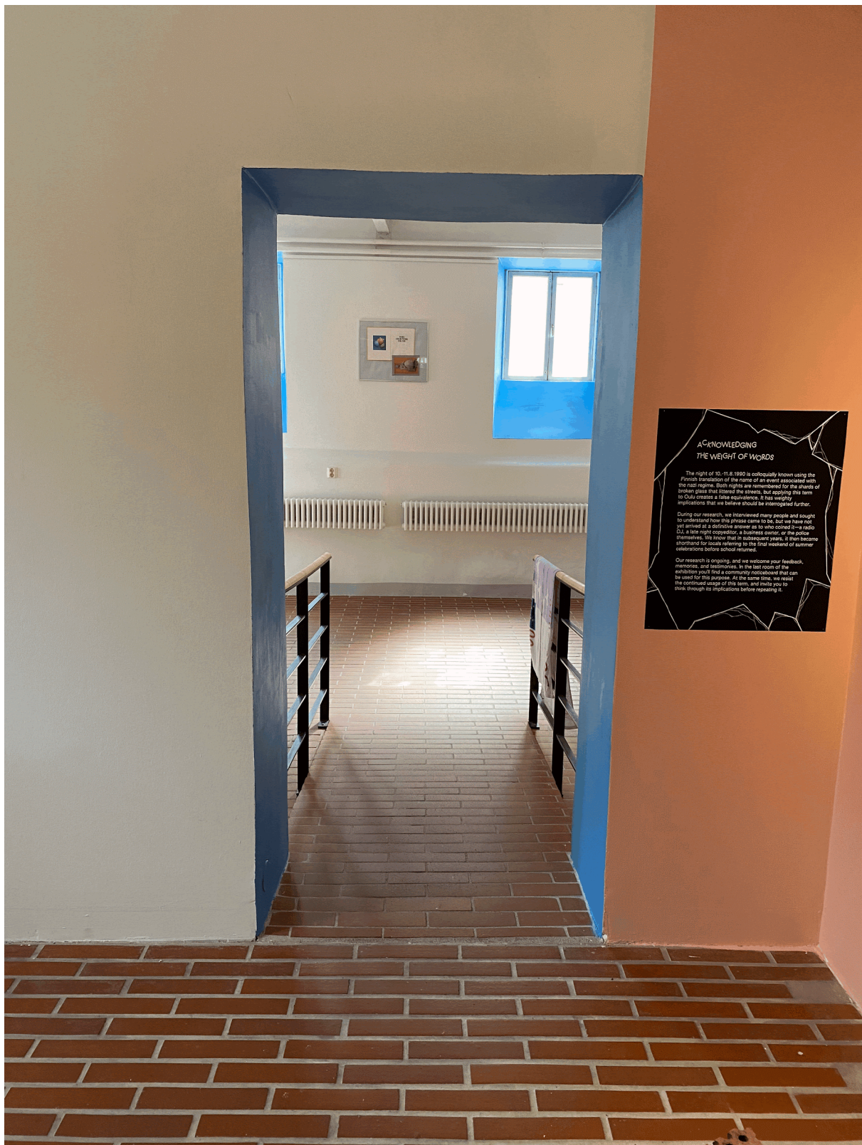
Doorway width to the back room (down a slope) 100 cm
